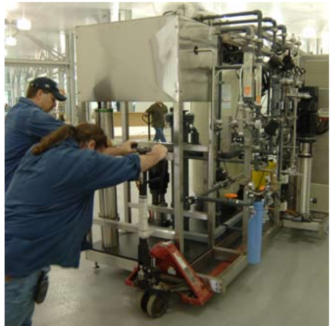
Installation of ultrapure water system in Andover, USA
