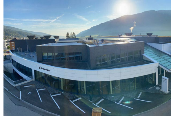
Operational improvements in Villeret, Switzerland
