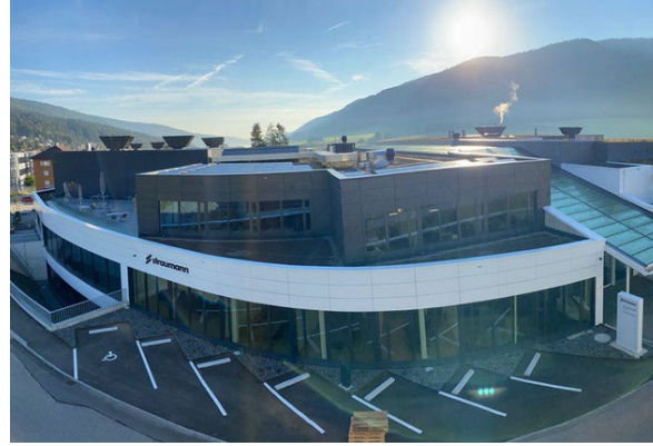
Operational improvements in Villeret, Switzerland
